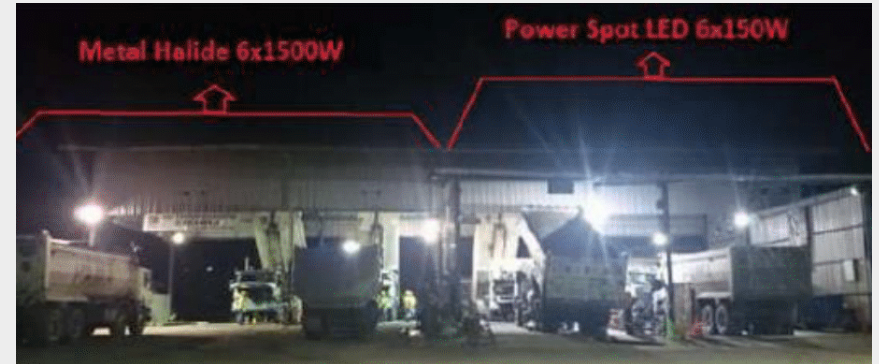
Workshop, 6 x 1500W Metal Halide vs LED Power Spot 6 x 150W
